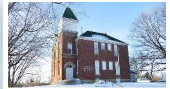
Elysian School Museum Closed: Under Renovation
